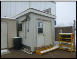
Foreman shack w/ contents
