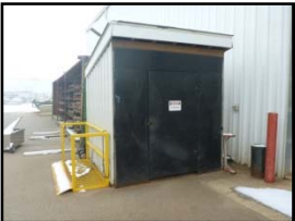
Storage shed for cylinders
